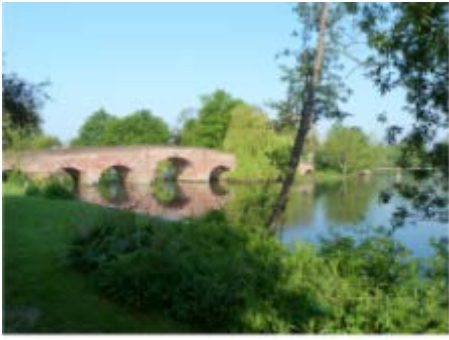
Bridge & Wharf May
