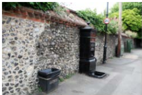
HS Pump_Deanery wall
